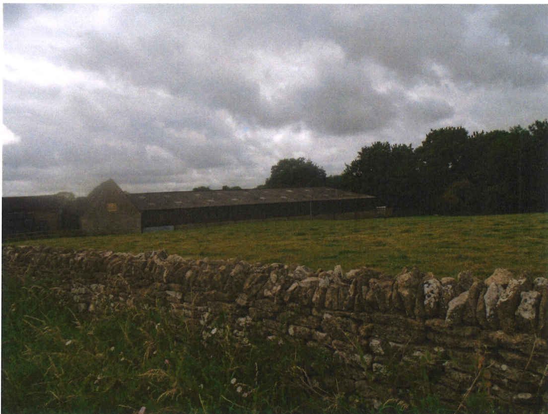
Southern buildings viewed from entrance drive
